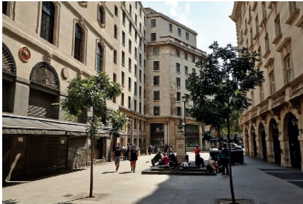
FIG 52 A view in Aldwych, with Herbert Baker's India House on the left.
