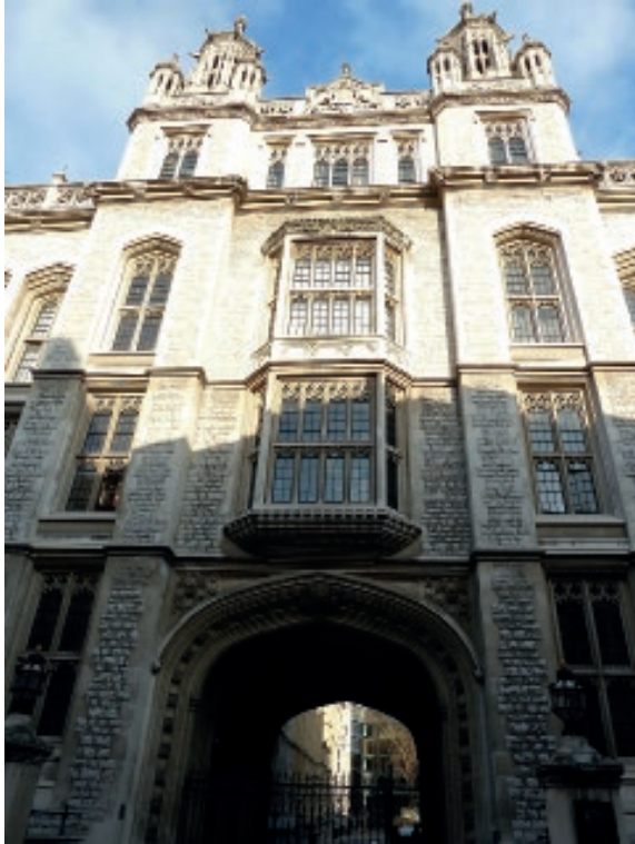
FIG 22 (LEFT) and 23 (BELOW) Two of the four campuses that King's College, London, occupies in and around the Strand: above, the old Public Record Office on Chancery Lane by James Pennethorne, now the Maughan Library; below, the reinforced concrete and plate glass of E D Jefferiss Matthews's Brutalist frontage to the Strand, which replaced a gateway by Robert Smirke.
