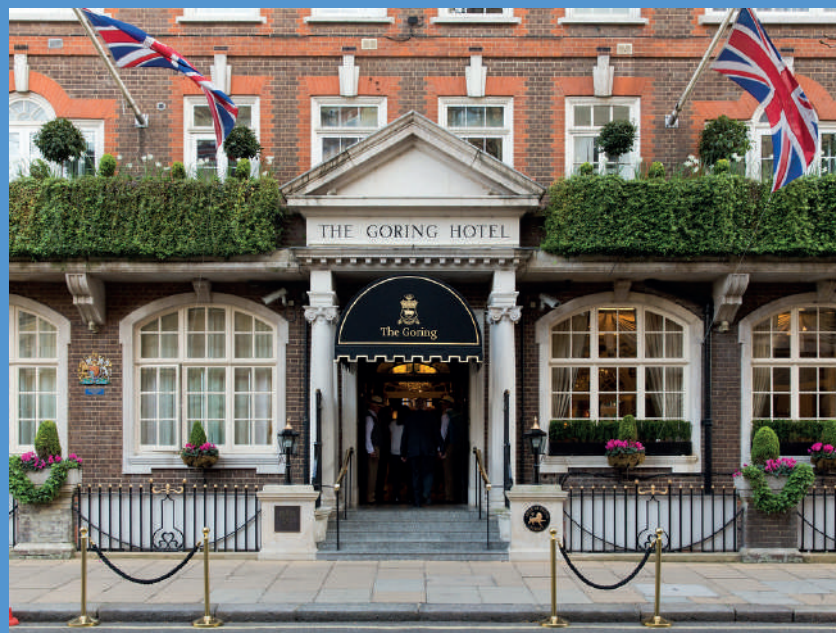
FIG 52 Entrance to the Goring Hotel.
