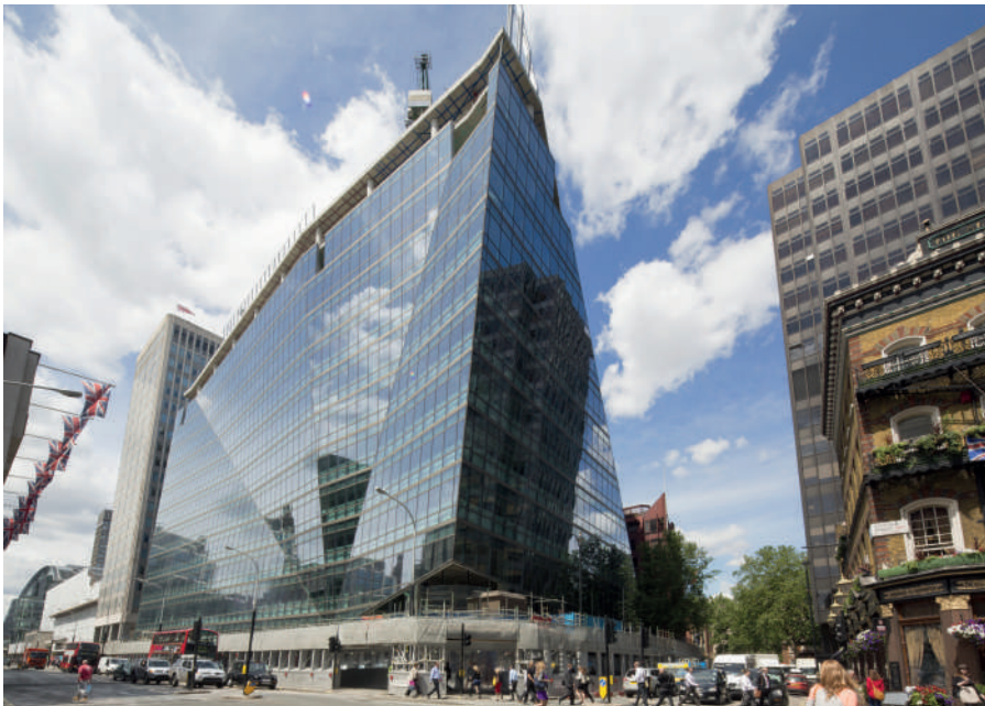
FIG 49 62 Buckingham Gate, completed in 2013.
