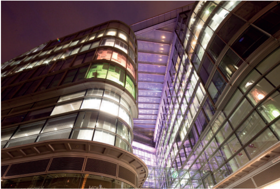
FIG 48 Cardinal Place, completed in 2006.
