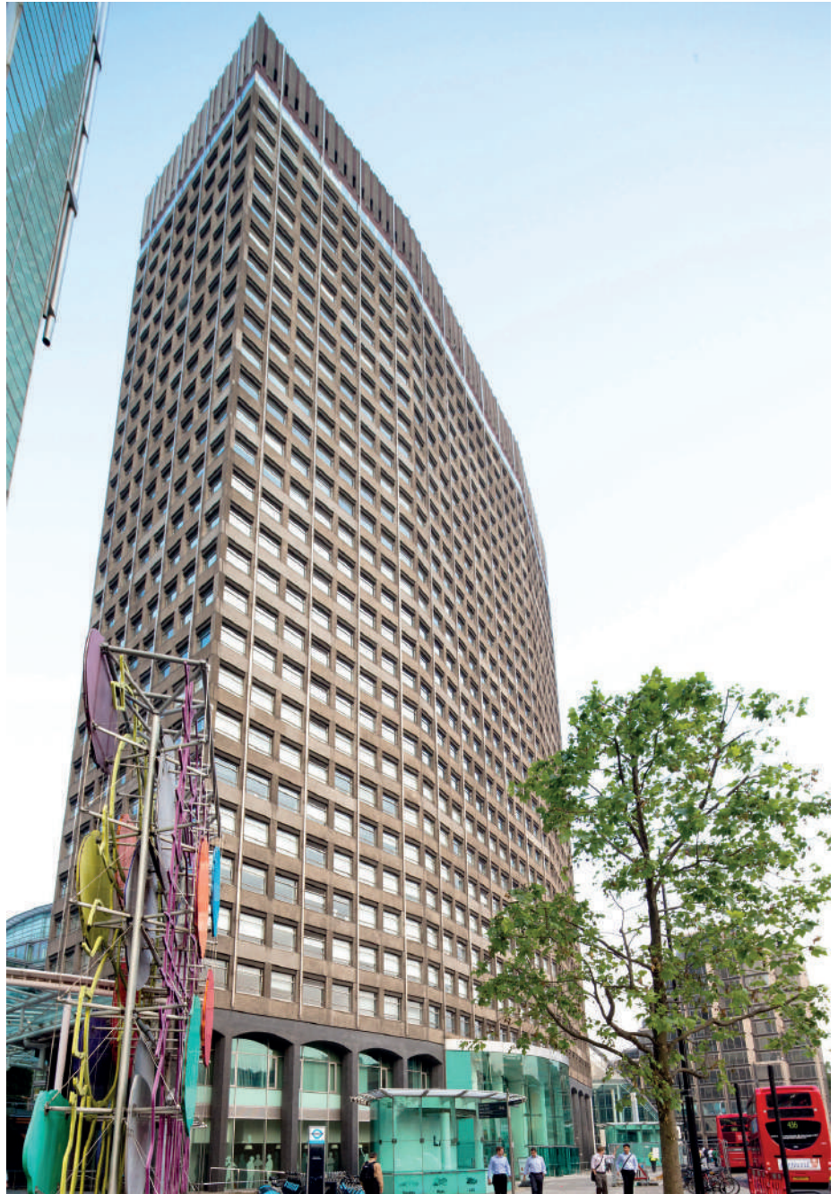
FIG 40 Portland House, completed in 1963.
