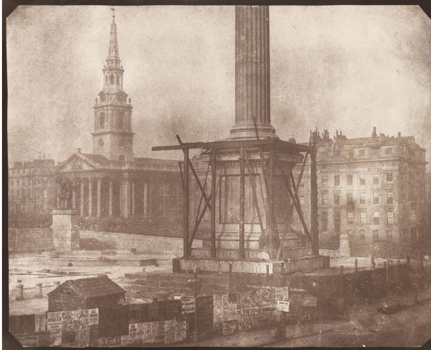
FIG 24 Nelson's column under construction, April 1844. Photograph by William Henry Fox Talbot (1800-1877).
